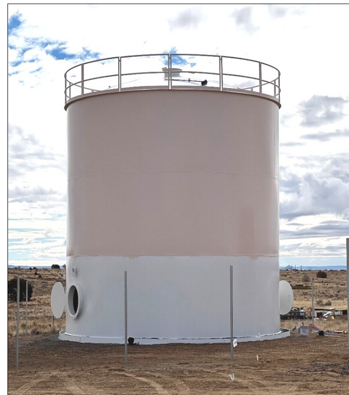
Hopi Tank 3 with coating almost complete
