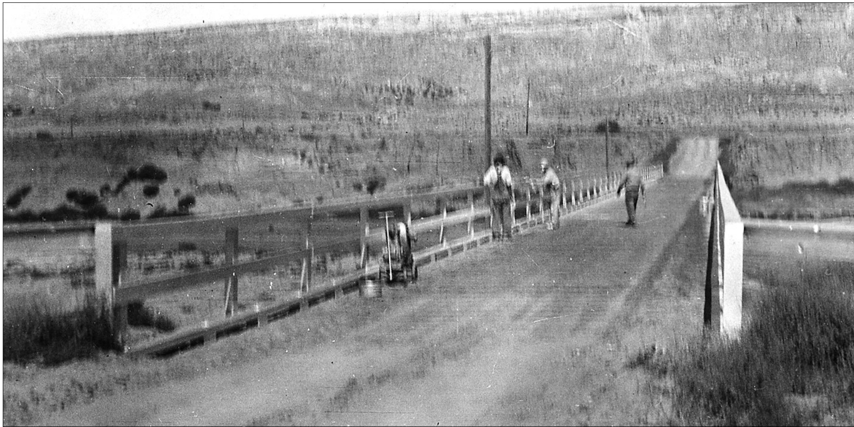
Notice how high original bridge stood from ground up, in comparison to today with clearance of only about four feet due to sediment built up
