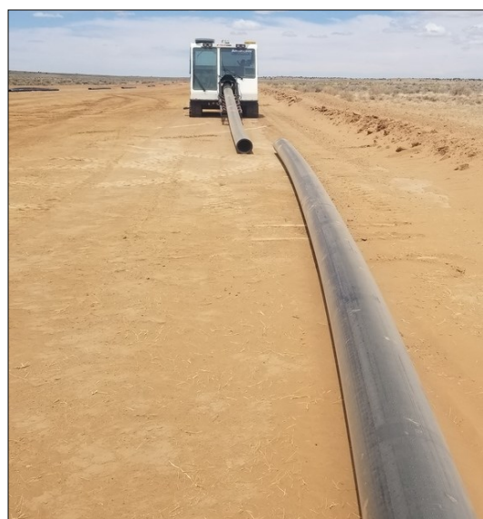
Project advances on schedule and is now near Wepo. Trenches are being dug, water pipes are fused together and laid in the ditches
