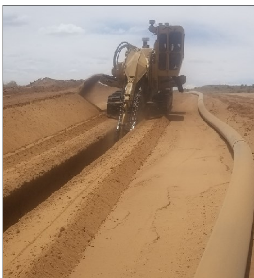
Project advances on schedule and is now near Wepo. Trenches are being dug, water pipes are fused together and laid in the ditches
