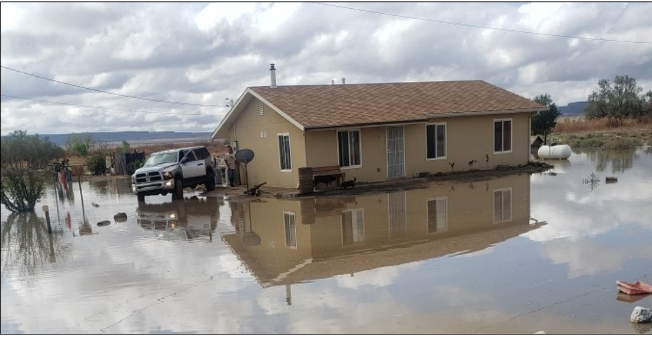
Family forced to evacuate from home after water spilled into their home
