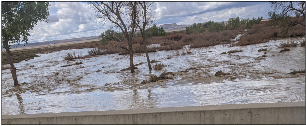
Flood waters gushing under Polacca Bridge SR 264 from East to West
