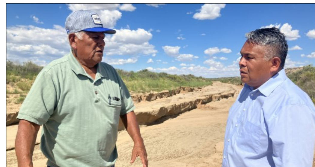
PHOTO: Hon. Council Delegate Kee Allen Begay, Jr. discussing with Ivan Sidney, Village Administrator for the First Mesa Consolidated Villages, potential avenues to have H60 improved while standing at a washed-out part.
