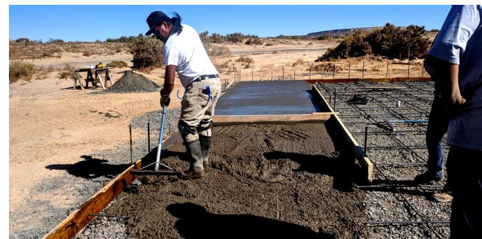
Volunteer Todd Siow lays foundation slab for skate ramp
