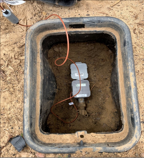
New Water Meters being Installed
