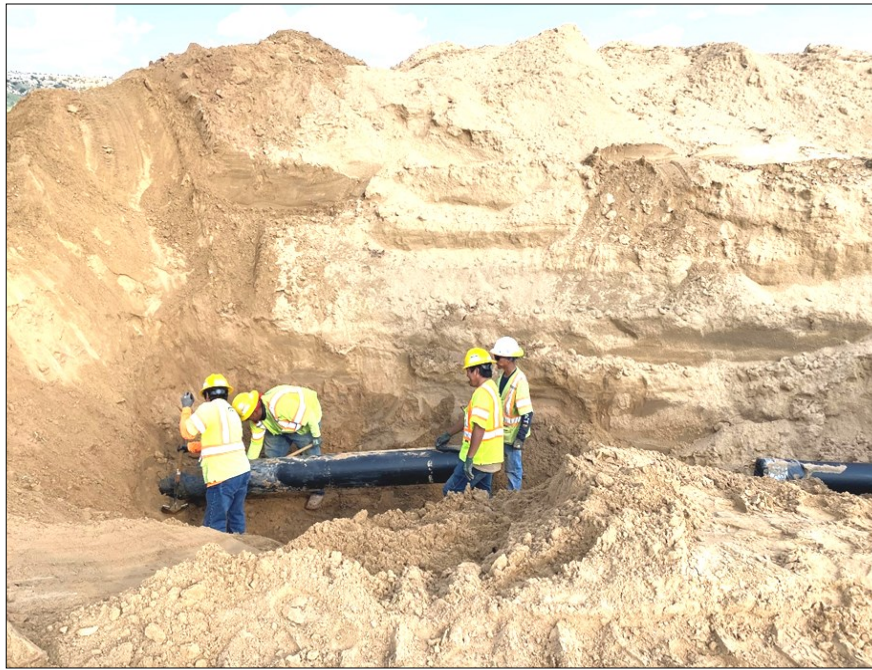
HAMP Pipeline installation along Route 8
