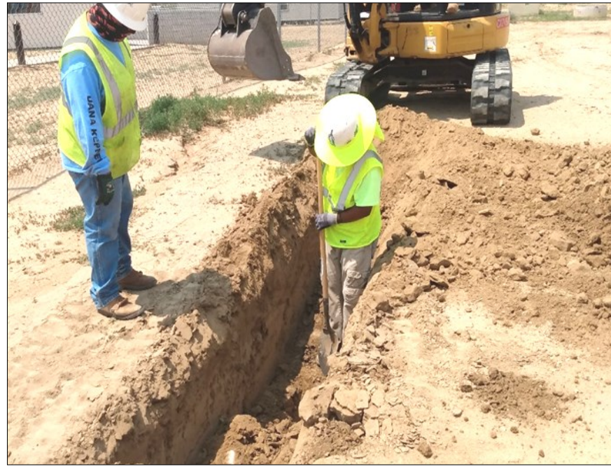
Contractor potholing for waterlines
