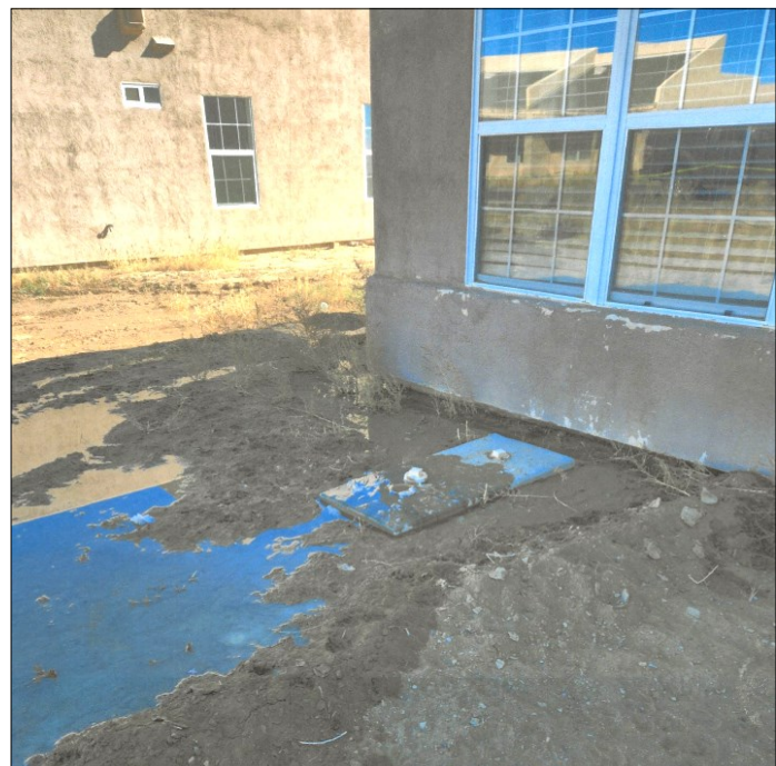
Wastewater Leakage flowing outside Walpi Housing
